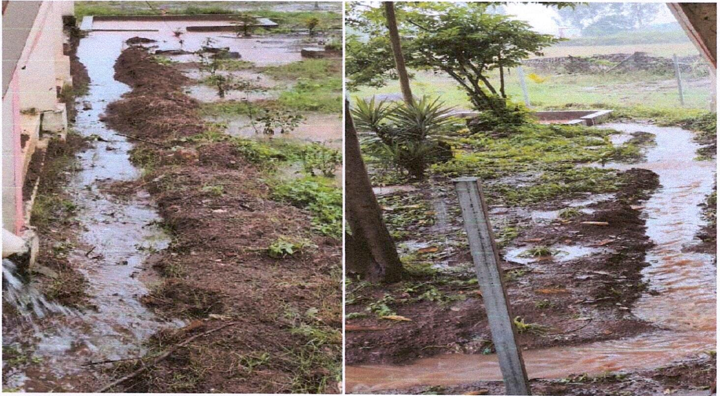
Rain water is conserved in to Percolation Pits
